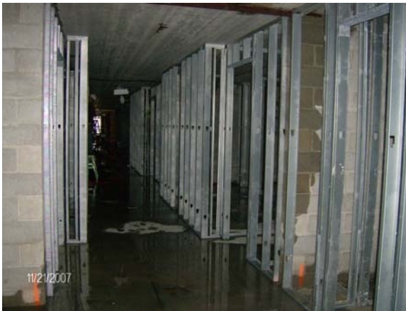
Hotel 3 rd Floor Interior Framing
