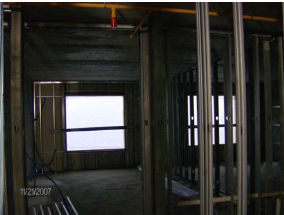
Hotel 2 nd Floor Interior Framing / Rough In
