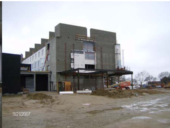
Hotel North Elevation
